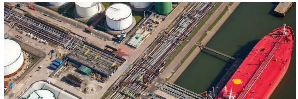
Loading & Offloading Services
